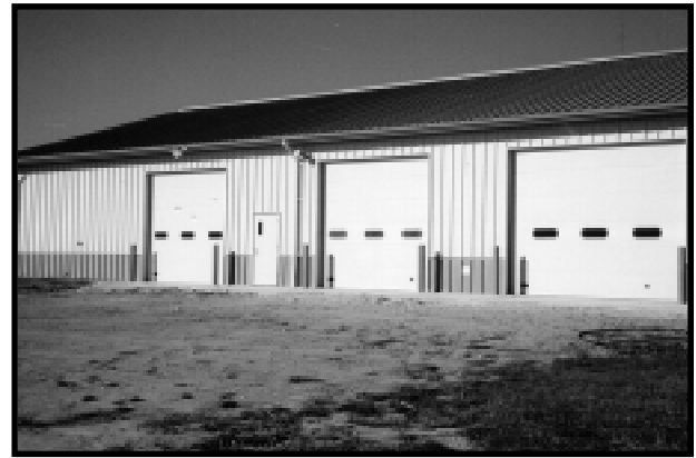
The vehicle storage and maintenance facility has unheated small vehicle storage in the bay at left. The maintenance bay in the center and the passenger loading area on the right are both heated.
